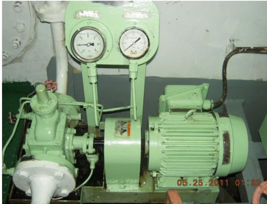
**Gambar 2.10 Pompa air pendingin**
