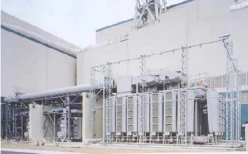
▲World's largest capacity three phase 1450MVA-500kV transformer for power stations and isolated phase bus which connects a power generator and transformer
