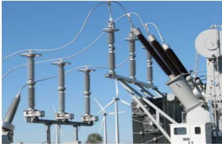
Gambar 2. 9 lightning arrester
