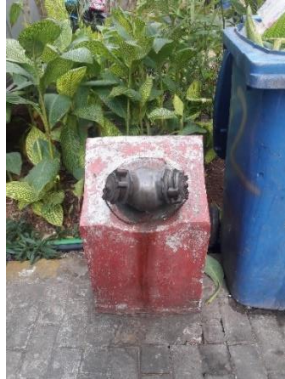
Gambar 4. 16 Gambar Siames Conection
