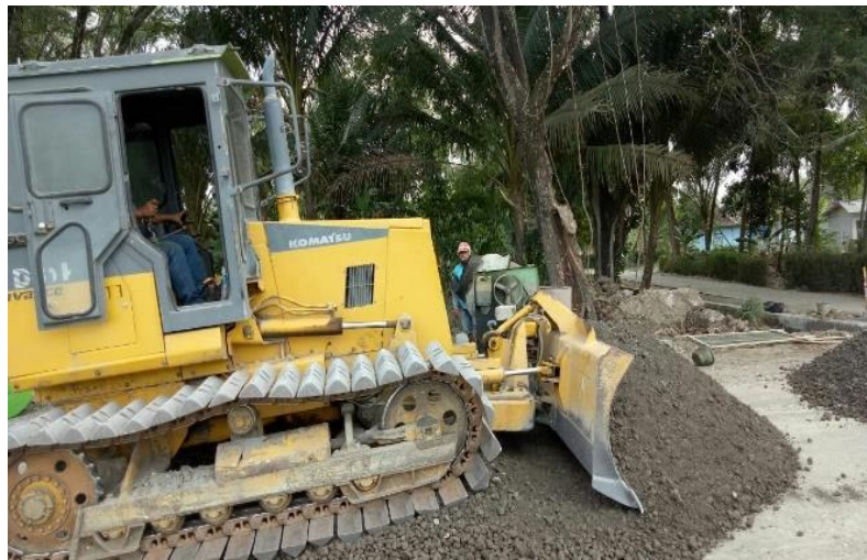
Gambar 4.3 Pekerjaan CTB ( Cemen Treatment Base )
