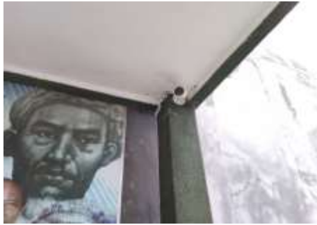
Gambar.4.8. CCTV Asrama Tahfidz
