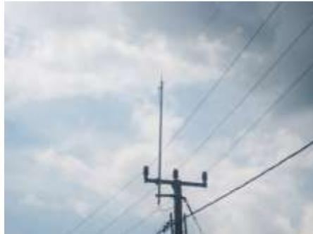
Gambar 2.13. Ground Steel Wire
