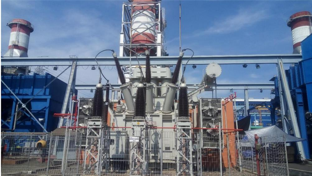
**Gambar 2. 8** *Generator Transformer* PLTGU Tambak Lorok Unit 2.2
