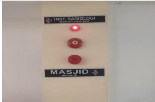
Gambar 2. 3 Fire alarm
