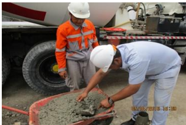
Gambar 4.4 Proses pengendalian mutu beton
