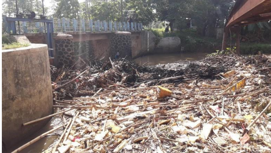
Picture 3. 1 The Picture of Koja Dam on 19 Desember 2018
