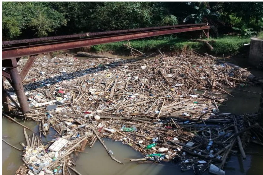
Picture 3. 2 The Current Condition of Koja Dam on 13 June 2019
