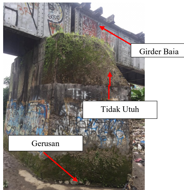
Gambar 4.18 Foto abutmen jembatan girder baja
