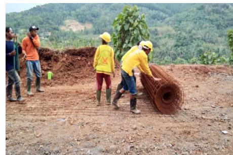
Gambar 9. Proses pemotongan besi wiremesh .
