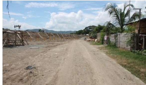
Figure 5. Mega Dike in Barangay Santiago
