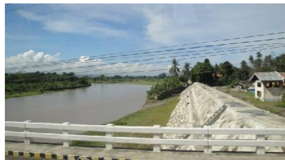
Figure 6. Riprapping of Mandulog River Bank
