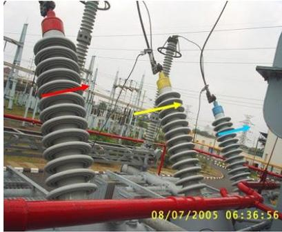
Gambar 2.8 Bushing Transformator
