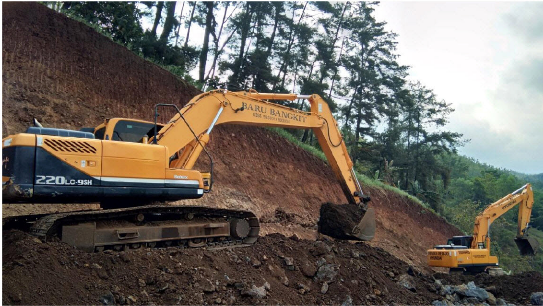
Gambar Proses Loading Tanah Galian
