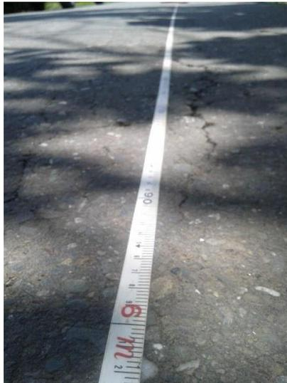
Gambar 2.27 Pengausan Agregat (*Polised Agregat*)
