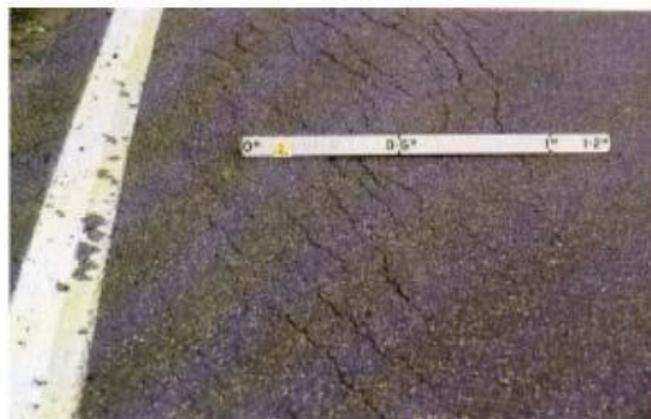
Gambar 2.37 Patah Slip (*Slippage Cracking*)
