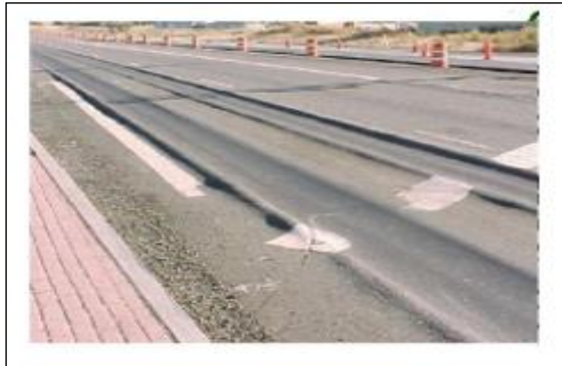
Gambar 2.31 Alur ( Rutting )
