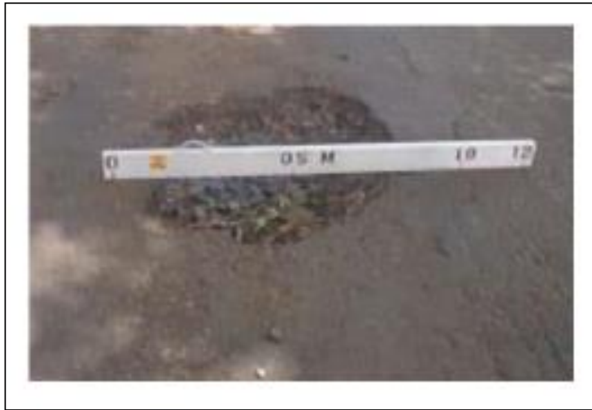
Gambar 2.27 Lubang ( Pathole )
