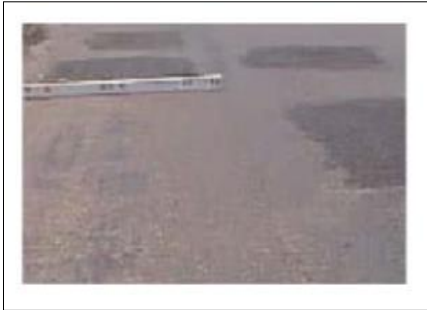
Gambar 2.23 Tambalan ( Patching and Utility Cut Patching )
