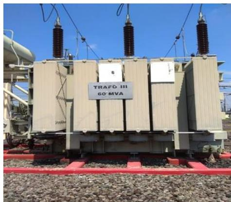
Gambar 2.1 Transformator 150 kV
