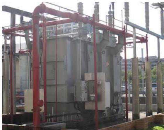
Gambar 2.4 Transformator Distribusi
