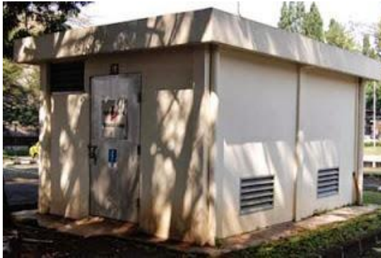
Gambar 2.2 Gardu Beton
