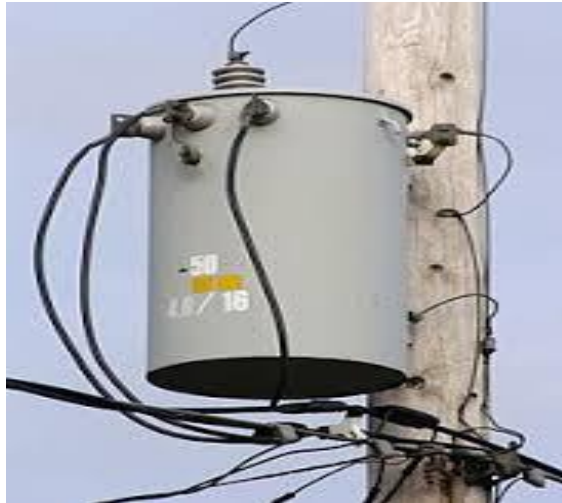
Gambar 2.6 Transformator 1 Pasa
