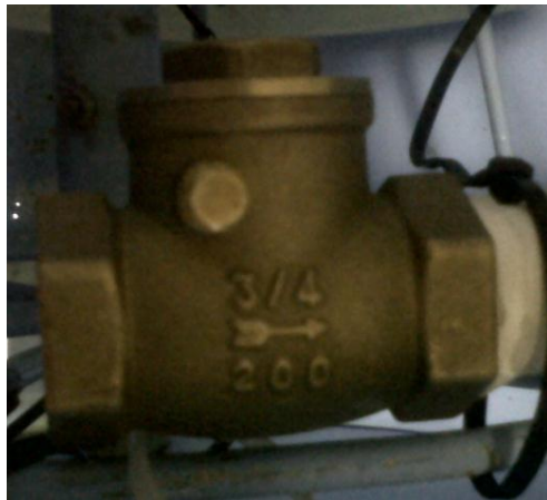
Gambar 3. 11. Check valve
