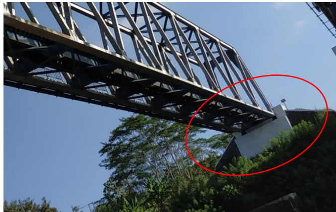
Gambar 4.53 Abutment Jembatan KA Mbeling II
