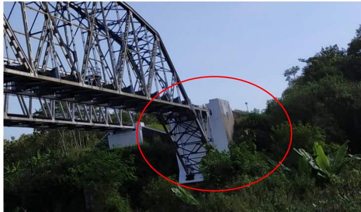
Gambar 4.50 Abutment Jembatan KA Mbeling I
