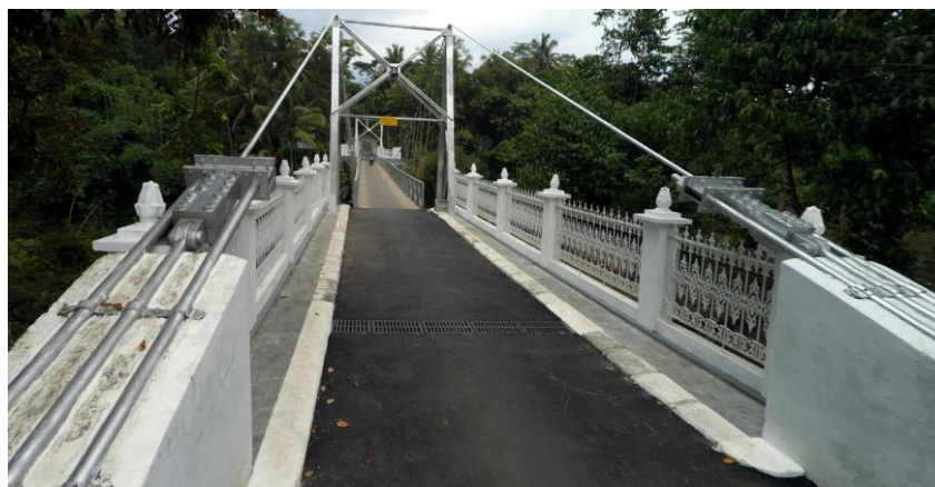
Gambar 4.37 Abutment jembatan Duwet
