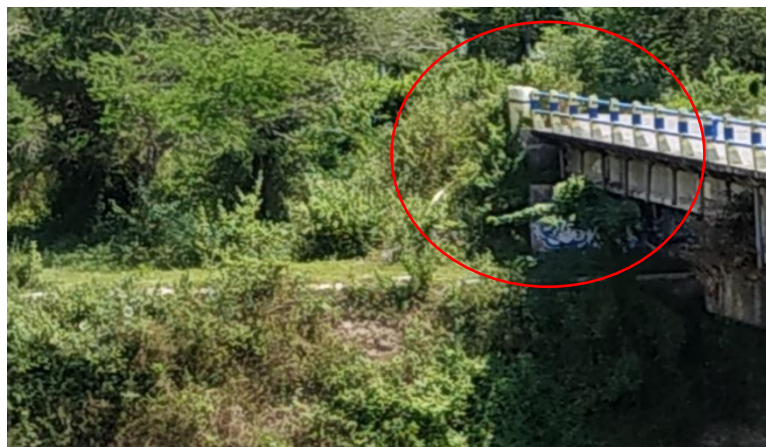
Gambar 4.33 Abutment jembatan Ancol
