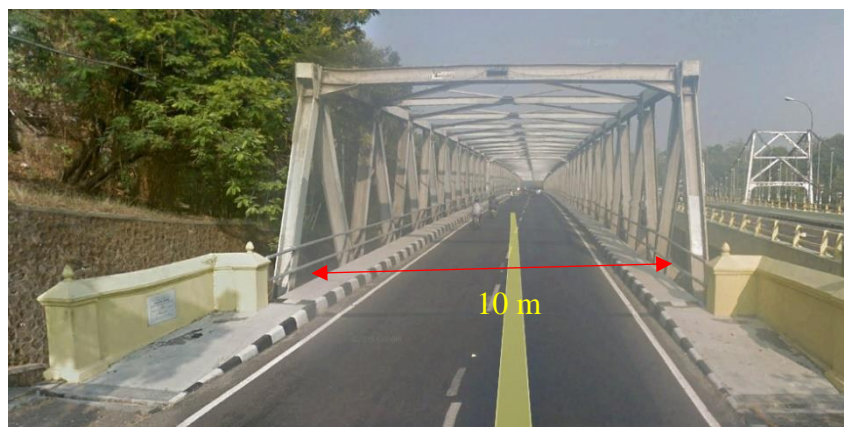
Gambar 4.58 Jembatan Bantar II (Baru) ( Google Earth, 2019 )
