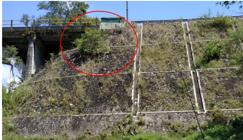
Gambar 4.29 Abutment jembatan Klangon
