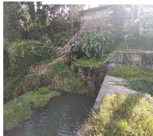
Dinding penahan tanah batu kali
