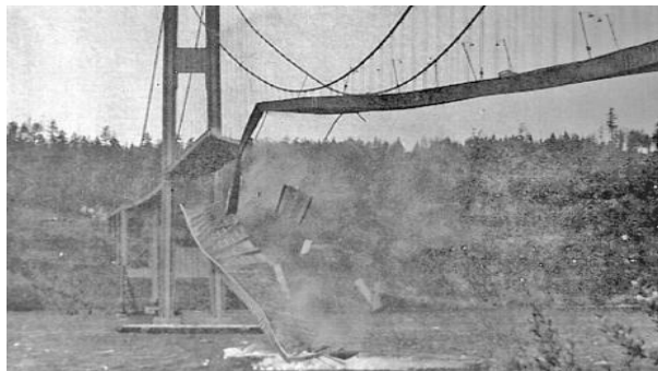
Gambar 2.8 Tipe keruntuhan zipper
