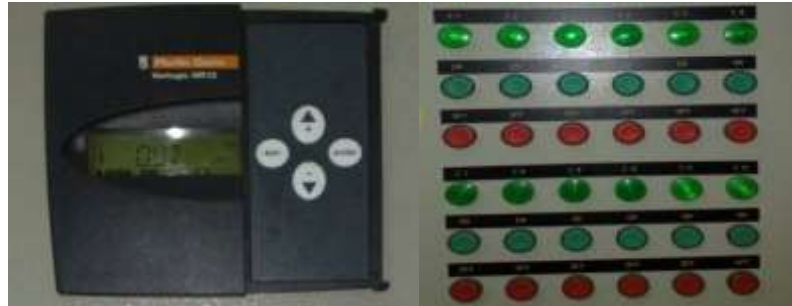
Gambar 2.22 Automatic Power Factor Regulator(APFR) (Sumber : Tarsin Saragih, 2011)
