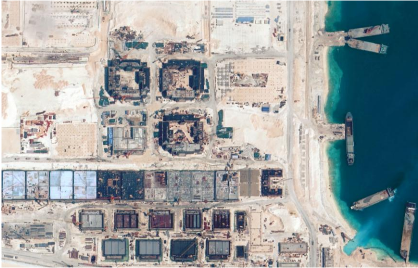
Figure 3.3 Building under construction on Fieri Cross Reef 114
