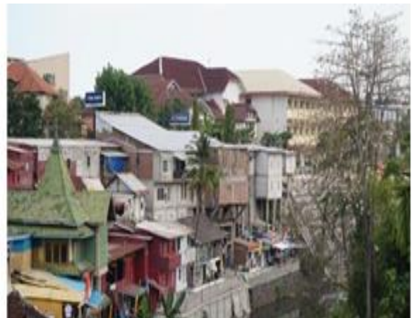
The real condition of public houses along the Sungai Code bank
