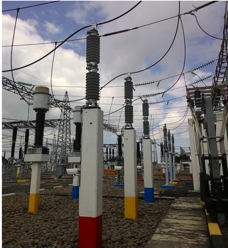
Gambar 5. Lightning Arrester
