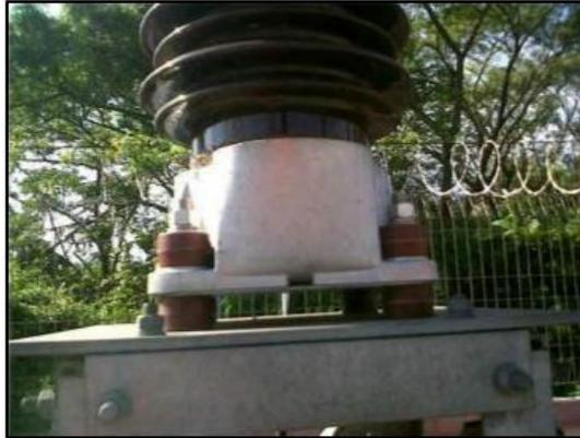
**Gambar 2.8** Insulator *Lightning Arrester*
