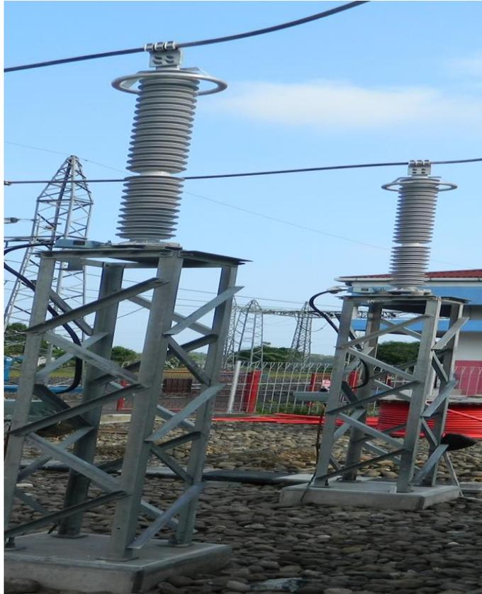
Gambar 2. 3 Lightning Arrester Gardu Induk Wates
