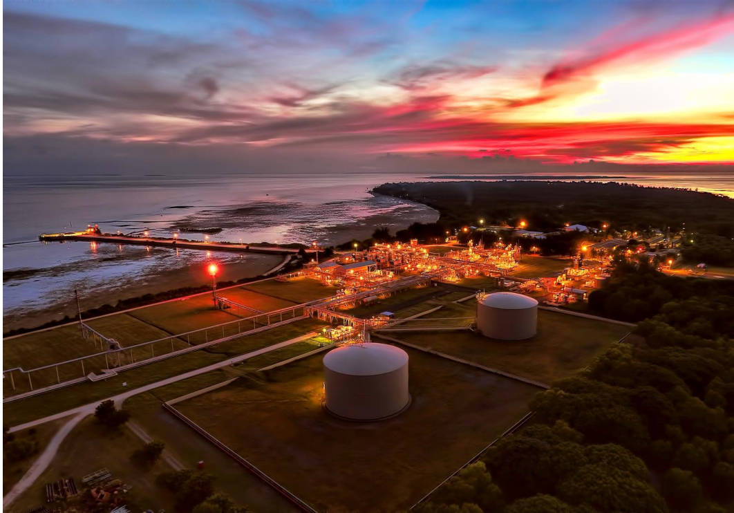
Lampiran 1. Gas Refinery Plant Kangean Energy Indonesia Ltd Pulau Pangerungan
