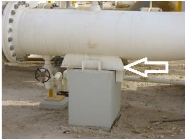
Gambar 5.7 Limit Stop/Stopper
