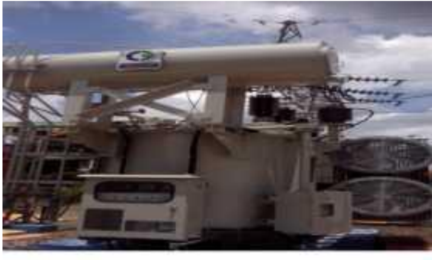
Gambar 2.2 Transformator daya
