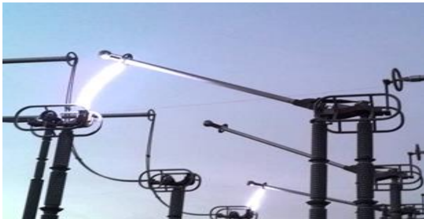
Gambar 2.7 Disconnection Switch (DS)
