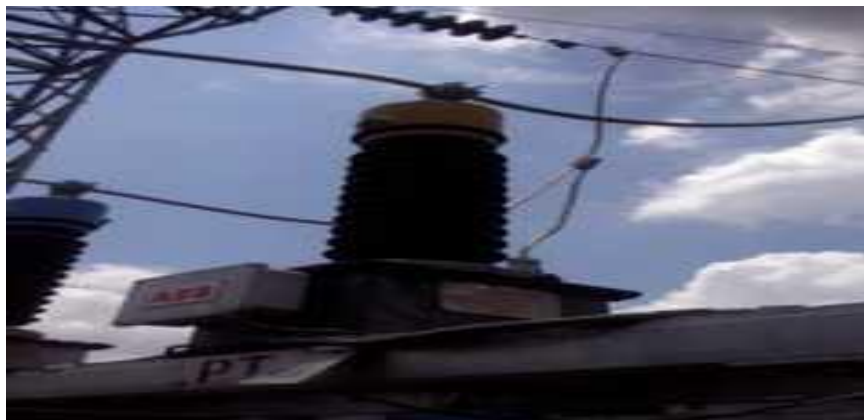
Gambar 2.5 Potential Transformator (PT)
