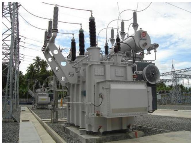
**Gambar 2. 6** Transformator Daya
