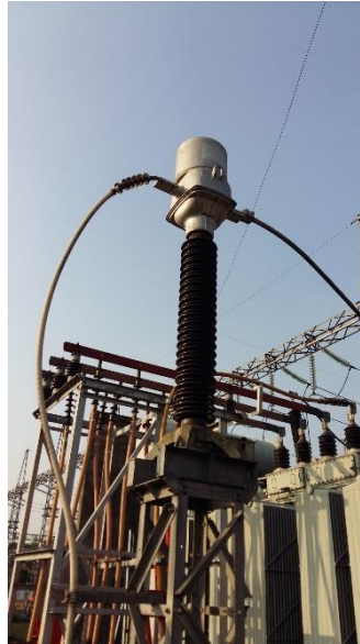
Gambar 2.3 Current Transformer
