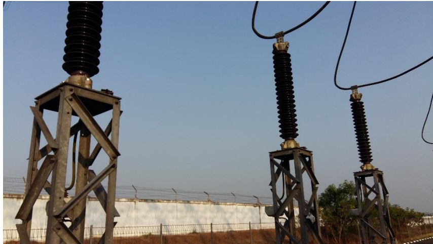
Gambar 2.4 Potential Transformer
