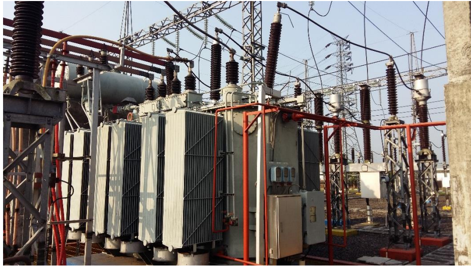
Gambar 2.2 Transformator Daya
