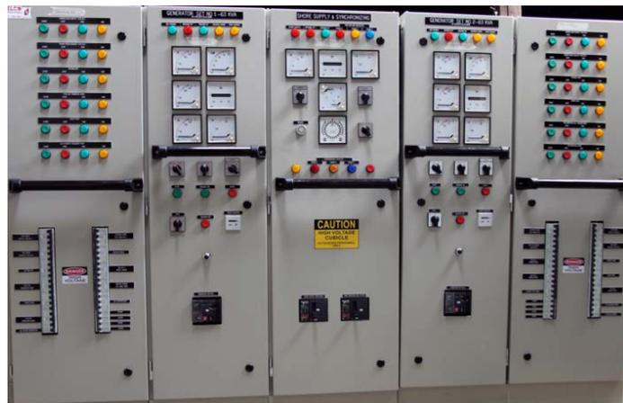
Gambar 2.8. *Low Voltage Main Distribution Panel* (LVMDP)
