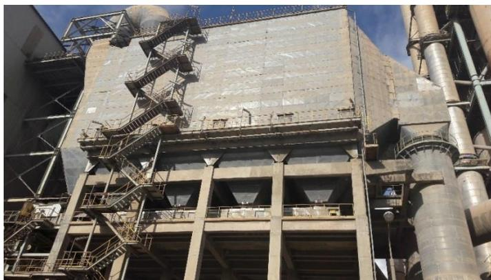
Gambar 2.1 *Electrostatic Precipitator*
