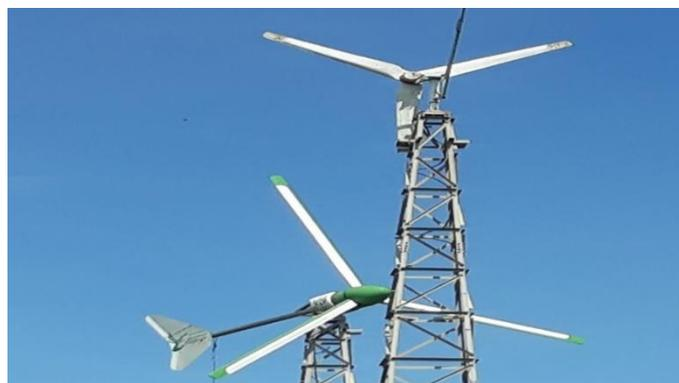
Gambar 2.9 Turbin Angin Sumbu Horizontal
