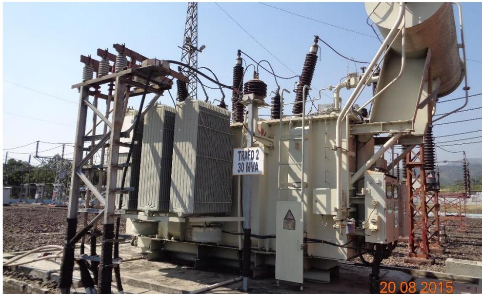
**Gambar 3.4** Transformator II berkapasitas 30 MVA 150/20 KV
