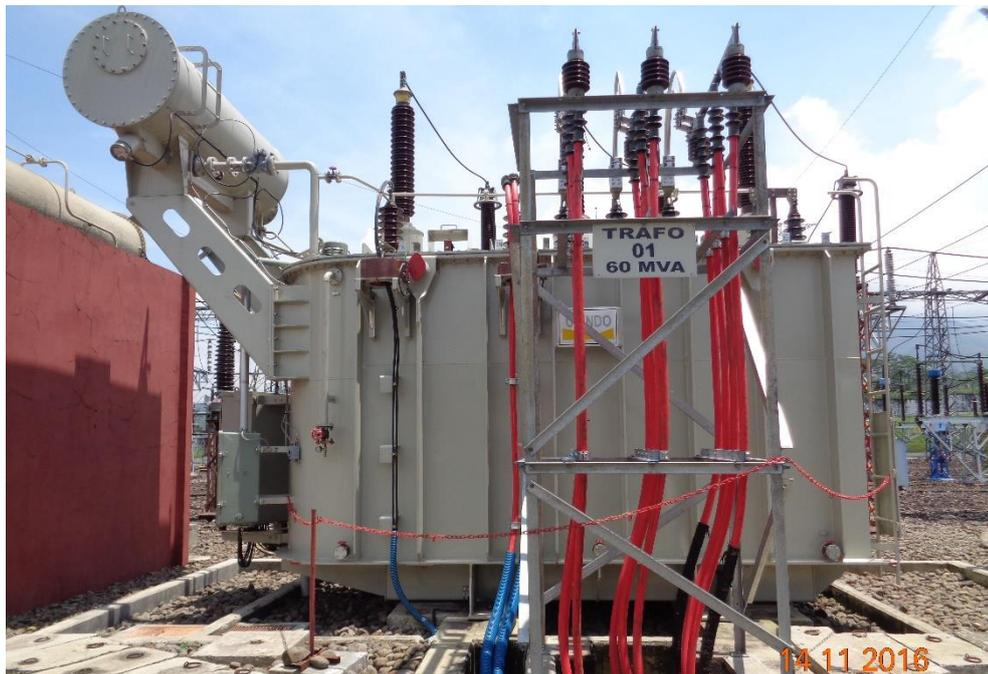
**Gambar 3.3** Transformator I (baru) berkapasitas 60 MVA 150/20 KV
