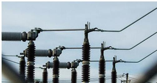
**Gambar 2.11** *Disconnecting Switch*
