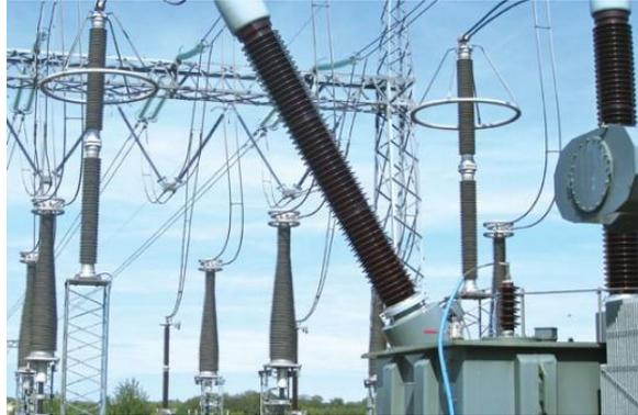
**Gambar 2.10** *Lightning Arrester*
