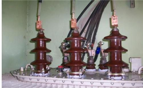
**Gambar 2.17** Bushing transformator
