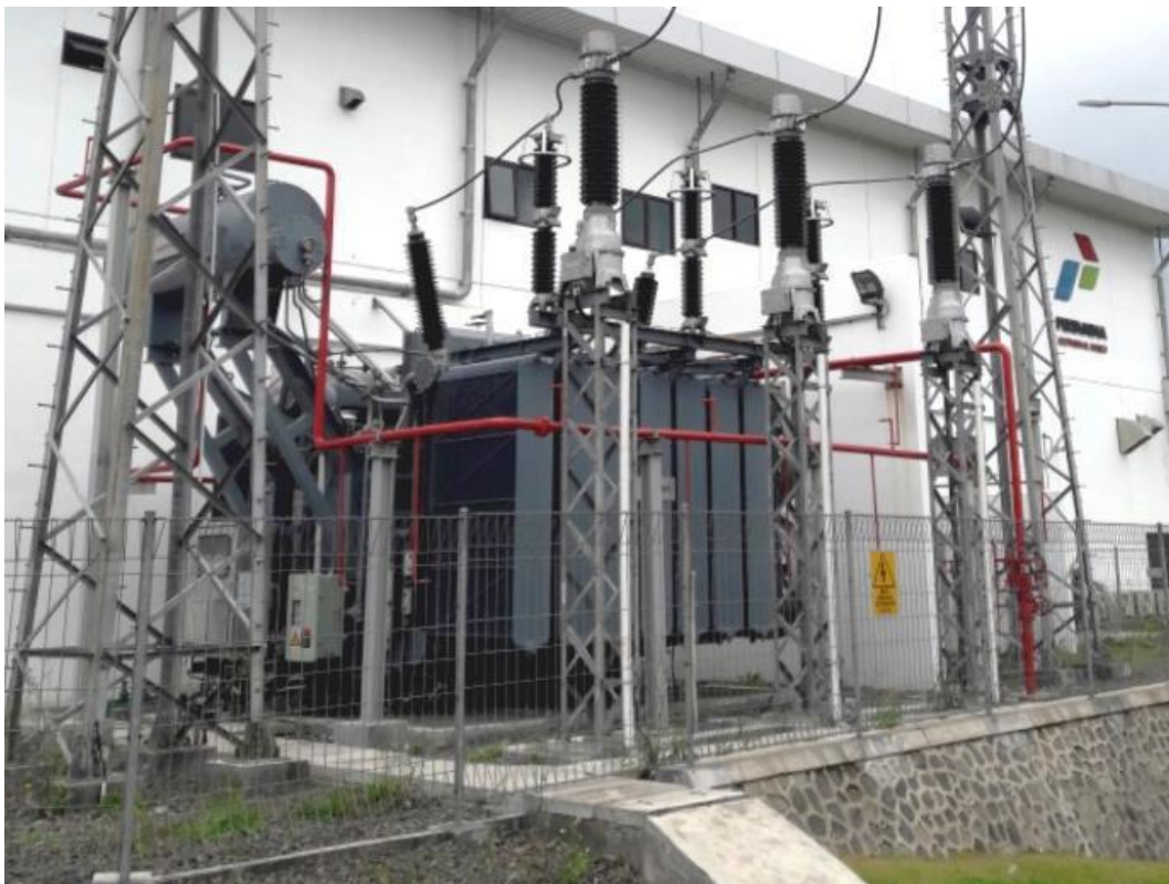
Lampiran 9. Transformator Daya PLTP KMJ Unit 5
