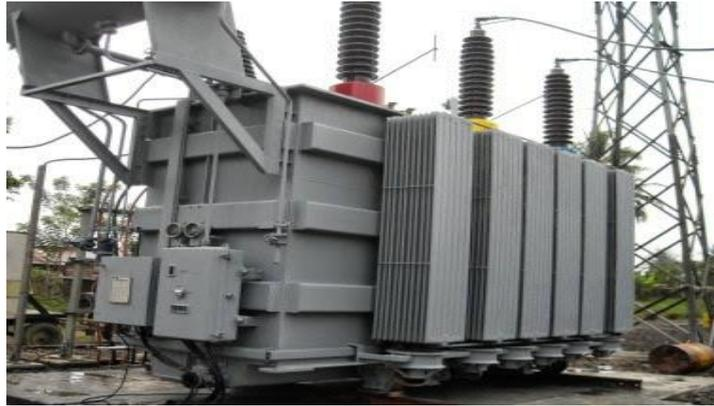
Gambar 2.2 Transformator daya
