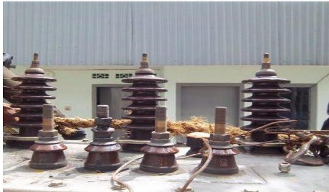
Gambar 2.13 Bushing Transformator
