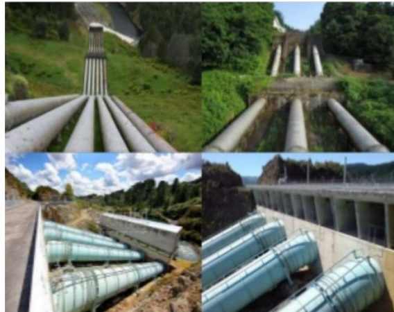
Gambar 2.15. Pipa Pesat (PENSTOCK)
