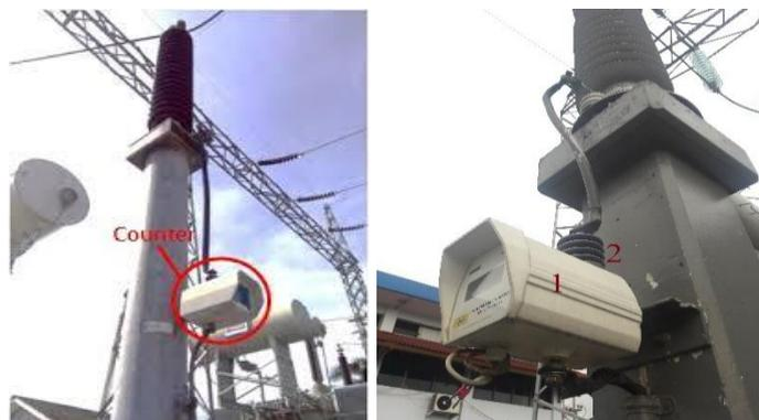
Gambar 2.23 *Discharge counter* arrester dan miliammeter (mA)
