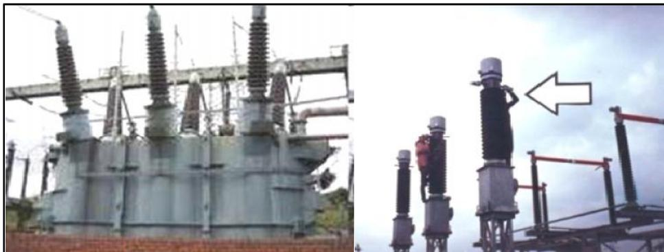
Gambar 2.6 Transformator Arus ( Current Transformer)
