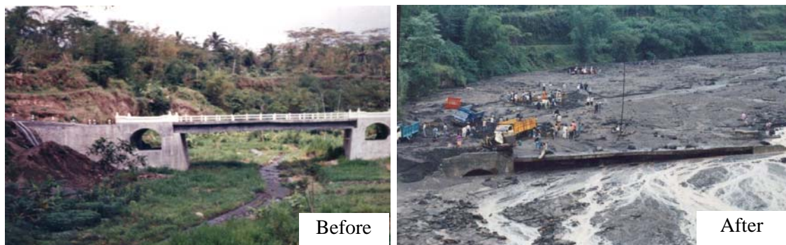
Photo 1.2 Kemiri Bridge on Boyong River after a debris flow in 1994 (Photo courtesy Adhy Kurniawan)
