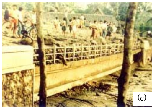
Photo 3.2 (a) Damages at a village on Krasak River after a debris flow in 1969, (b) Damages on houses in a village near Krasak River after a debris flow in 1976, and (c) A bridge condition on Putih River after a debris flow in 1984 (Photo courtesy Adhy Kurniawan)
